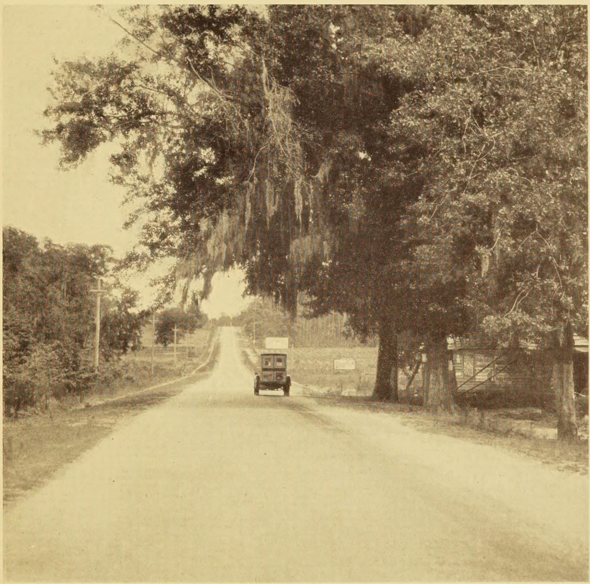
A BITUMINOUS SURFACE TREATMENT OF A LIME ROCK ROAD IN FLORIDA
